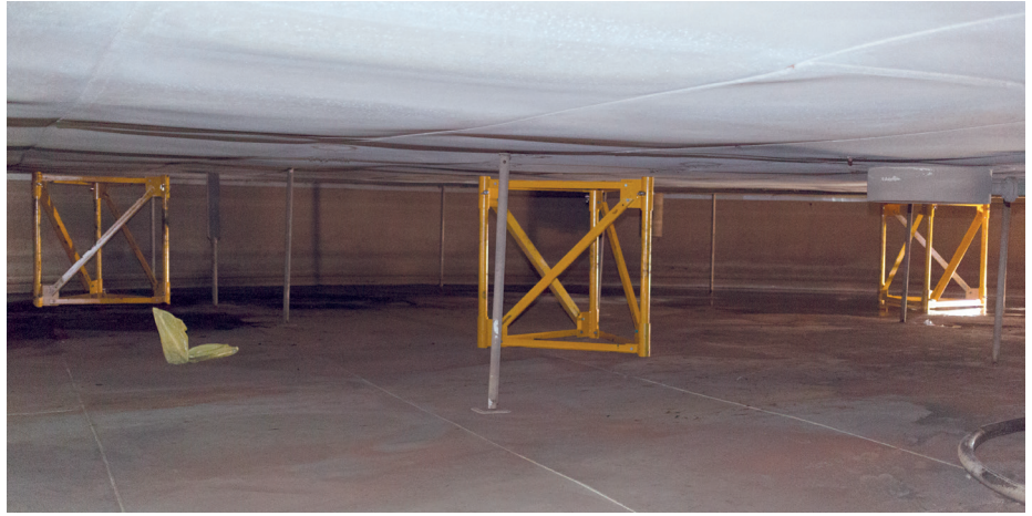
The Delta P Cribbing Tower being utilised during a tank inspection at Alon USA Refinery's facility in Big Spring, Texas
